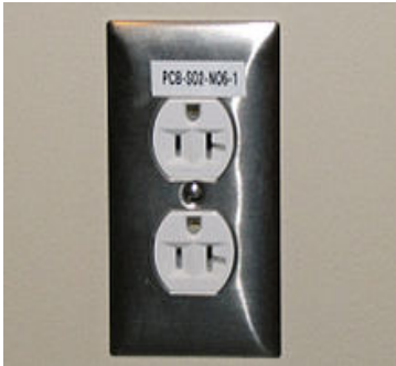
NEMA 5-20 – Standard ground outlet with 20 amp capability
